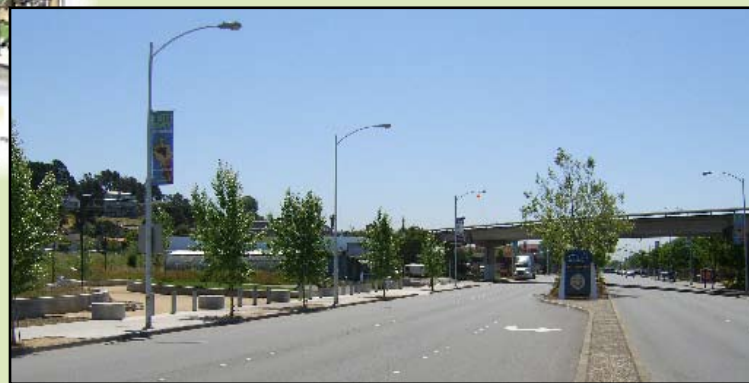
INSTALLED BAXTER CREEK STREET FRONTAGE AND NEW WELCOME SIGN
