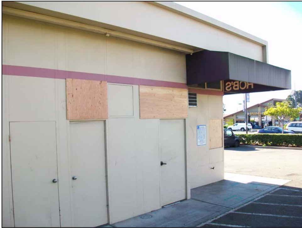
10192 San Pablo Avenue/SR 123. North façade detail, view to the southwest. 12/27/2016.
