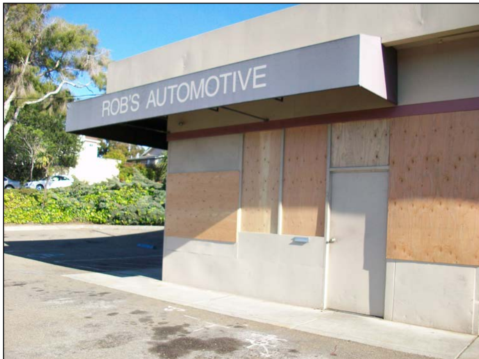
10192 San Pablo Avenue/SR 123. Main façade detail, view to the north. 12/27/2016.
