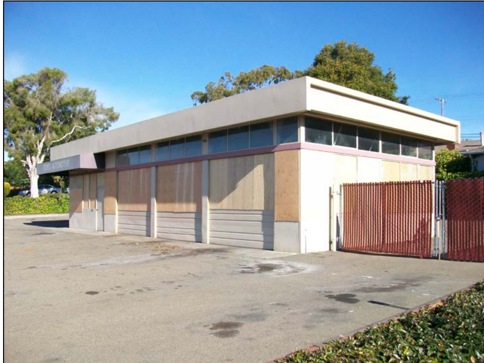
10192 San Pablo Avenue/SR 123. Main façade, view to the north. 12/27/2016.
