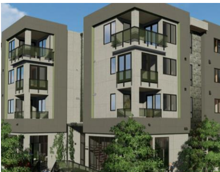
Under Construction: 10300 San Pablo Ave.
